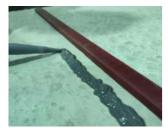
Apply the sealant to the prepared concrete surface by a slow uniform motion. To do this, squeeze a sufficient amount of sealant out of the tube. Apply the sealant in a strip with no gaps in the middle of the seam of the concrete element. If the concrete surface has any roughnesses, the sealant amount must be sufficient for aligning them.
