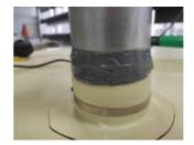
For additional sealing, it is recommended to treat the edge of the membrane with the TECHNONICOL LOGICFLEX polyurethane sealant. For this purpose, if necessary, remove excess swelling sealant and apply the TECHNONICOL LOGICFLEX PU sealant in such a way that it closes the upper clamp and connects to the pipe base, forming a hermetic lock.
