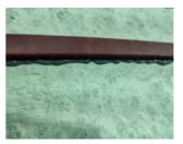
For fixation of a LOGICBASE IC-SP 20x10 bar, lay the polymer bar over the sealant applied in the middle of the joint.
