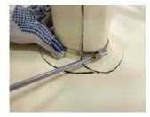
Upon welding the membrane, install a clamp with the corresponding diameter, which should securely fix the membrane on the pipe.
